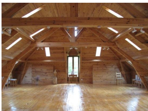
Yoga room - before
